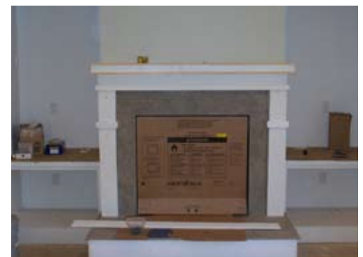
Custom Cabinets and Fireplace in progress.
